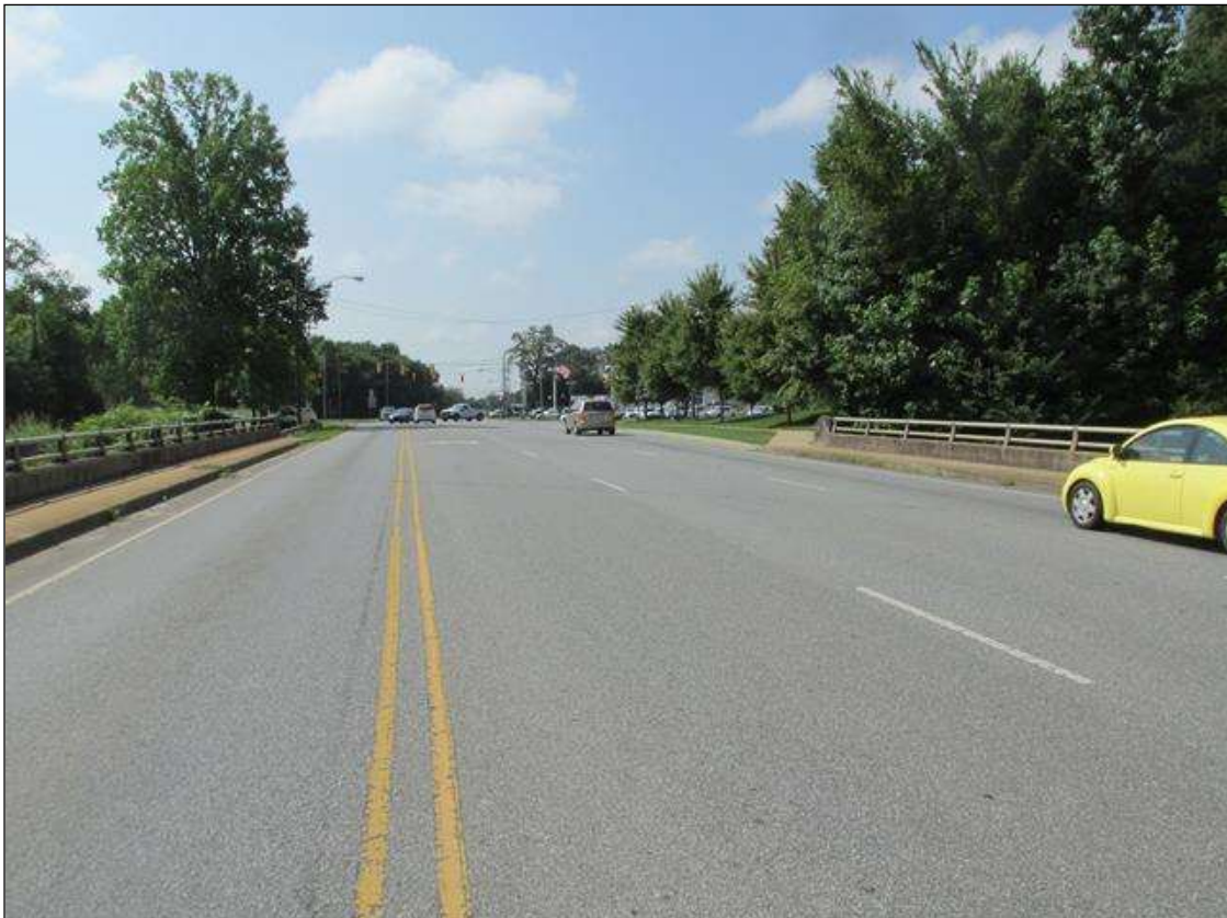
GUARDRAIL LOOKING SOUTH
