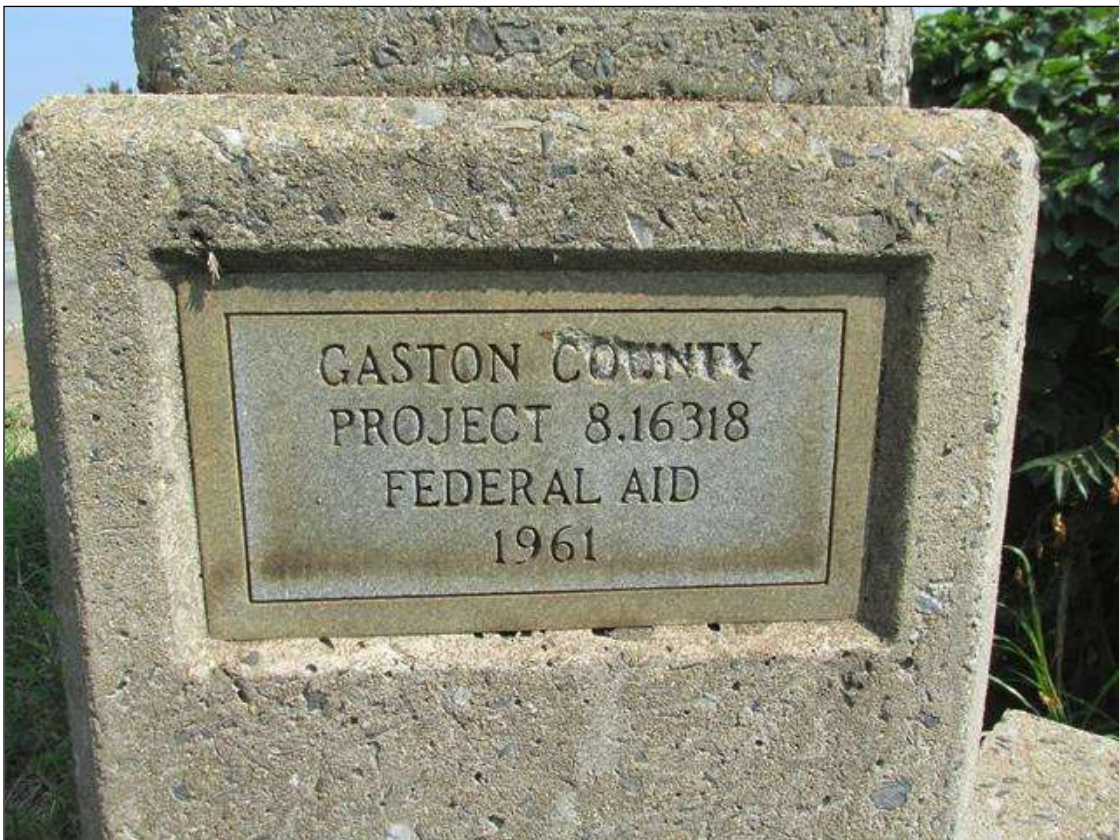
DATA PLATE, SOUTHEAST CORNER
