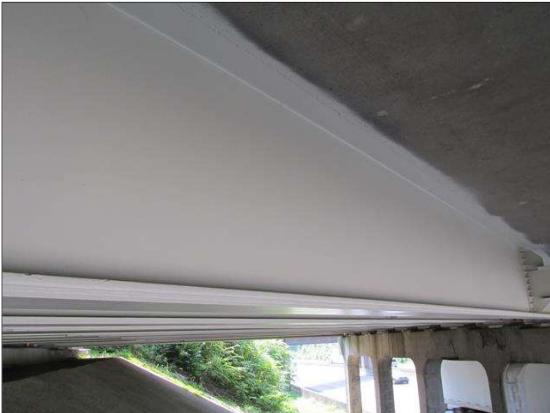
BEAMS PAINTED SINCE LAST INSPECTION.
