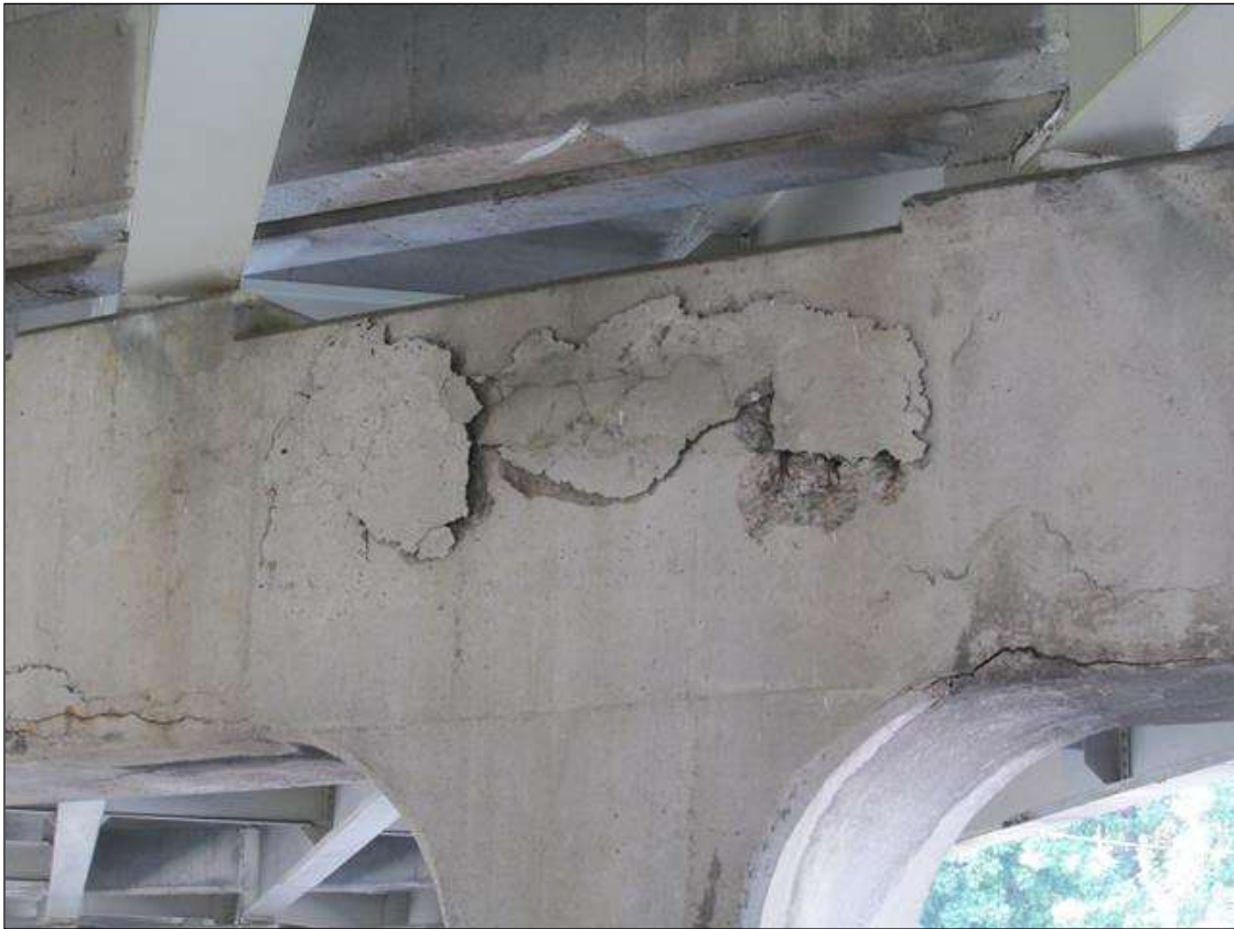
SPALLING WITH RESTEEL EXPOSED, BENT 3 CAP, ABOVE C2, APPROX 6'L X 2'H
