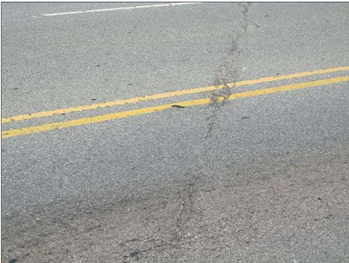
JOINT 1 CRACKED AND OPEN UP TO 1", FULL WIDTH
