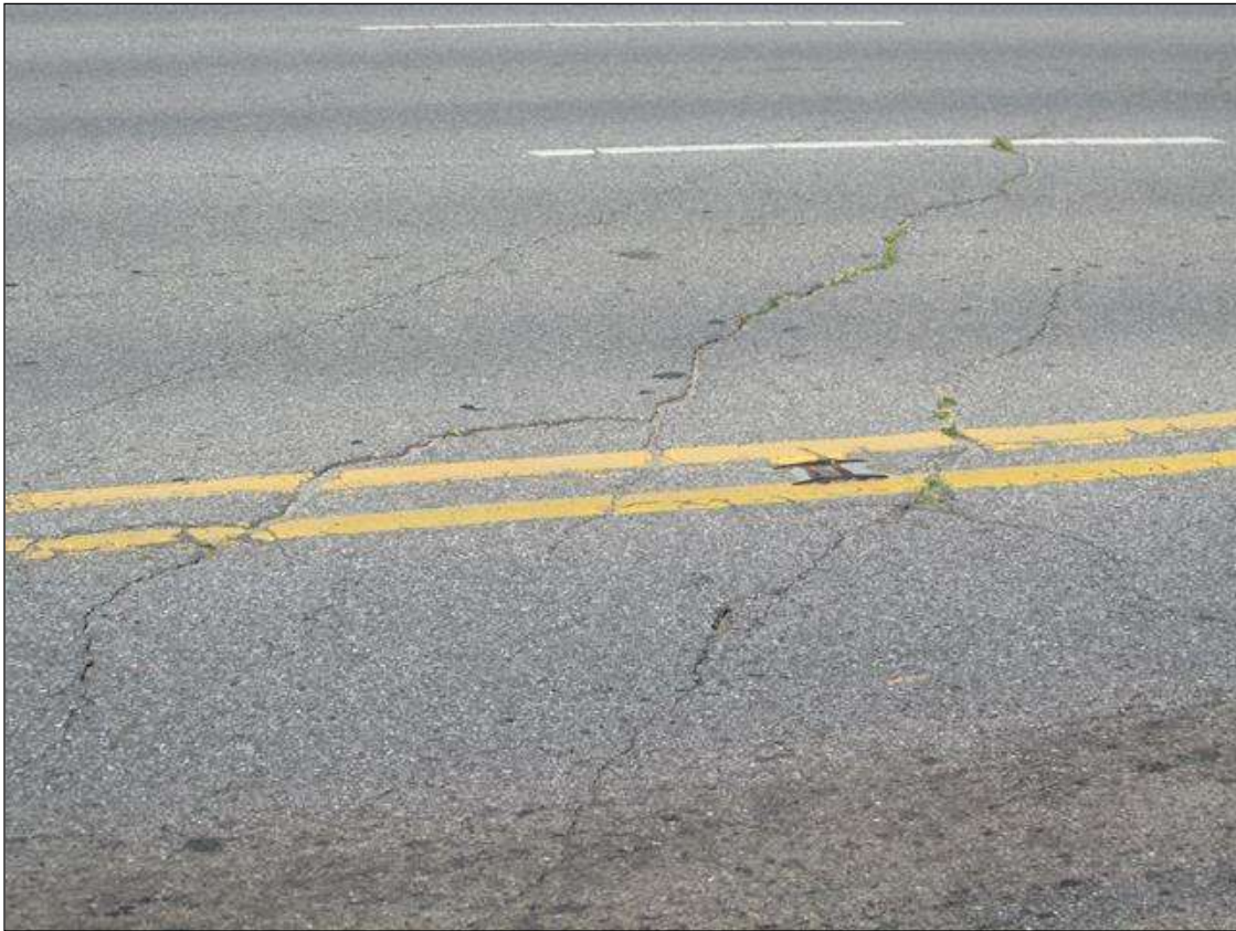
SOUTH APPROACH AWS CRACKED AND SUNKEN UP TO 0.5" FULL WIDTH.
