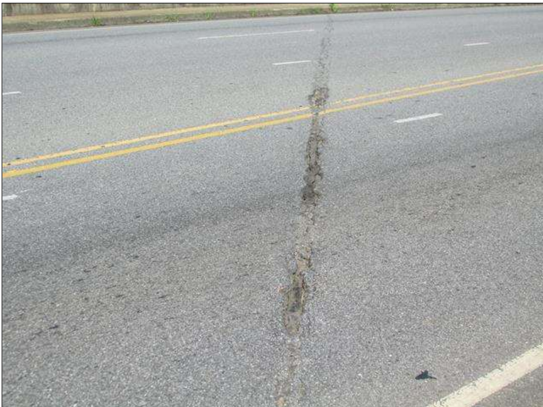
JOINT 3 CRACKED FULL WIDTH, OPEN UP TO 4"W X UP TO 2"D
