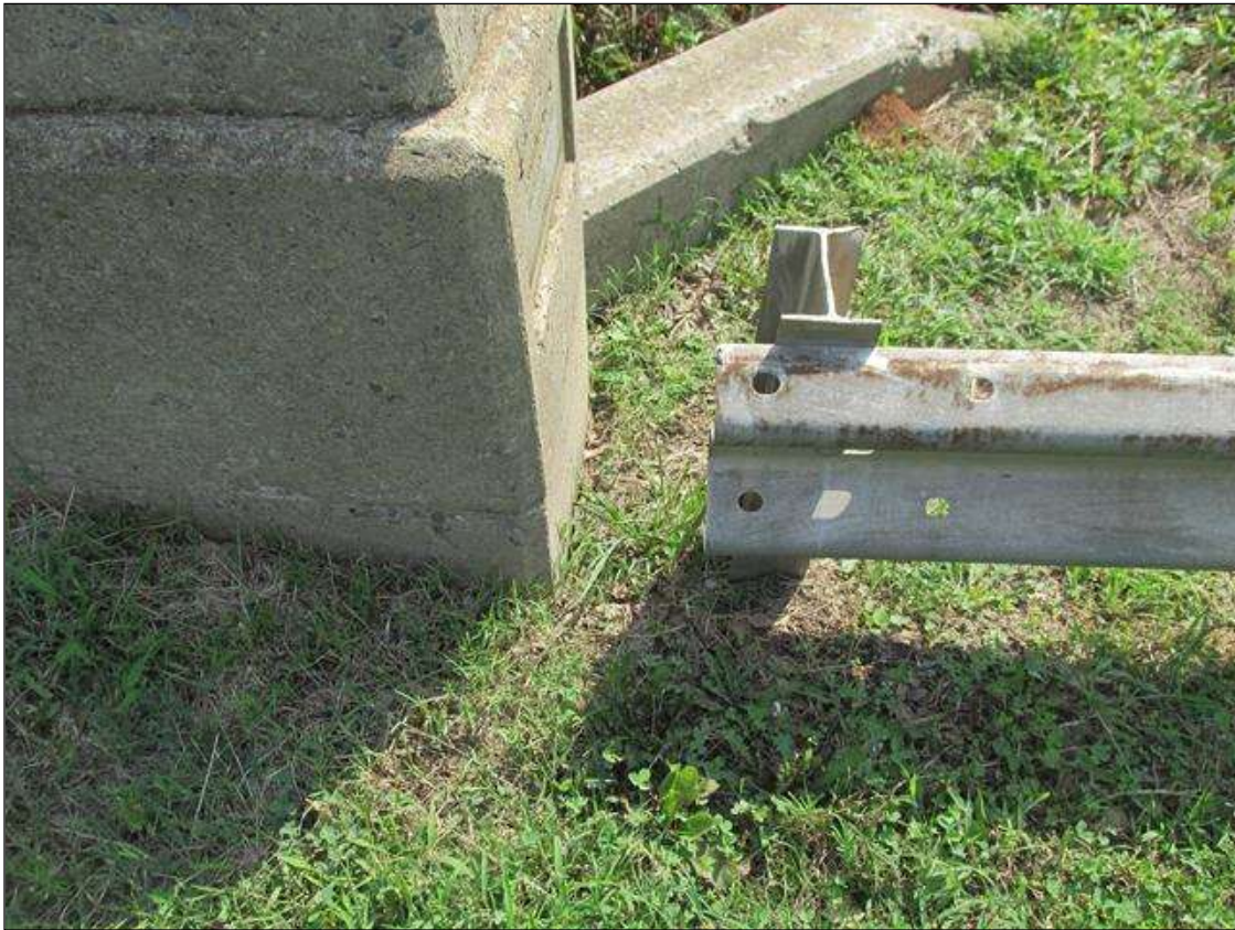
GR NOT CONNECTED, SOUTHEAST & NORTHWEST CORNERS
