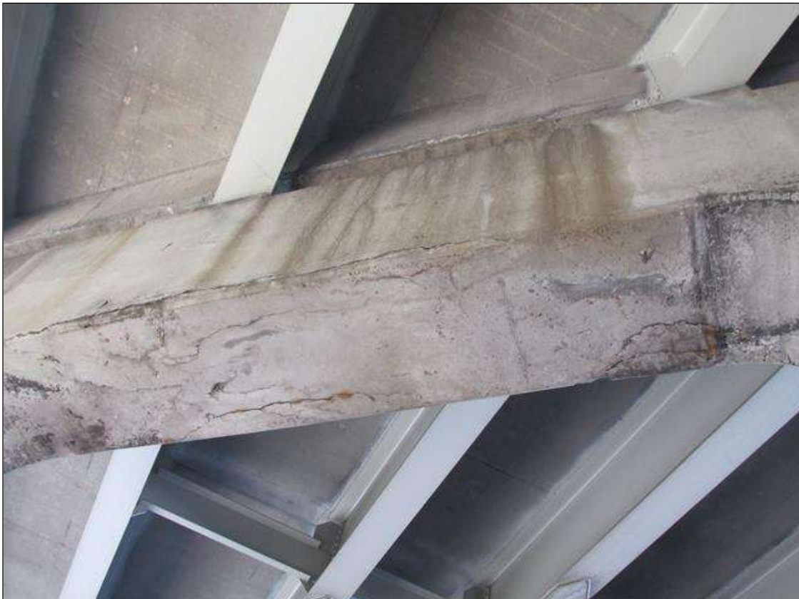
SPALLING WITH RESTEEL EXPOSED, BENT 3 CAP, BOTTOM SIDE OF CAP, BTWN C3-4, APPROX 8'L X 4'W
