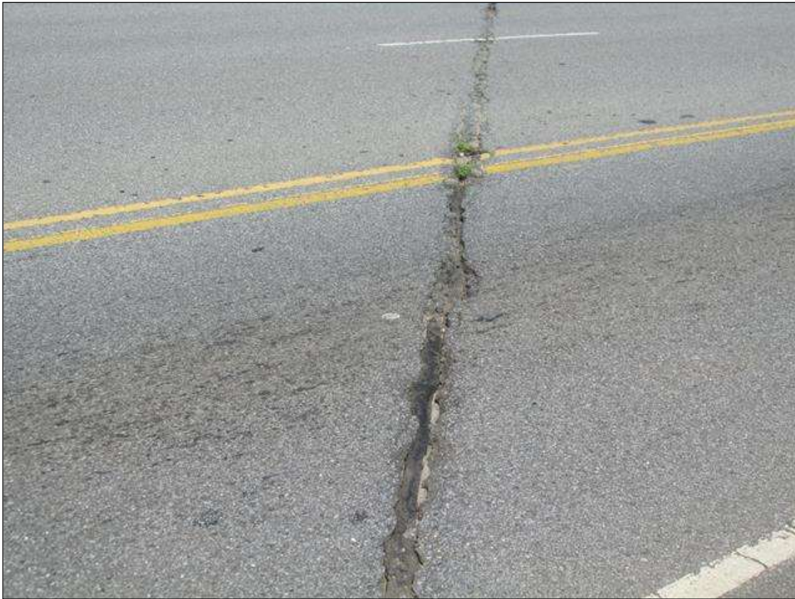
JOINT 2 CRACKED FULL WIDTH, OPEN UP TO 2.5"W X UP TO 2"D
