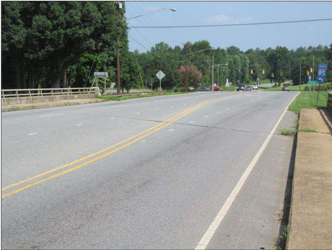
GUARDRAIL LOOKING NORTH
