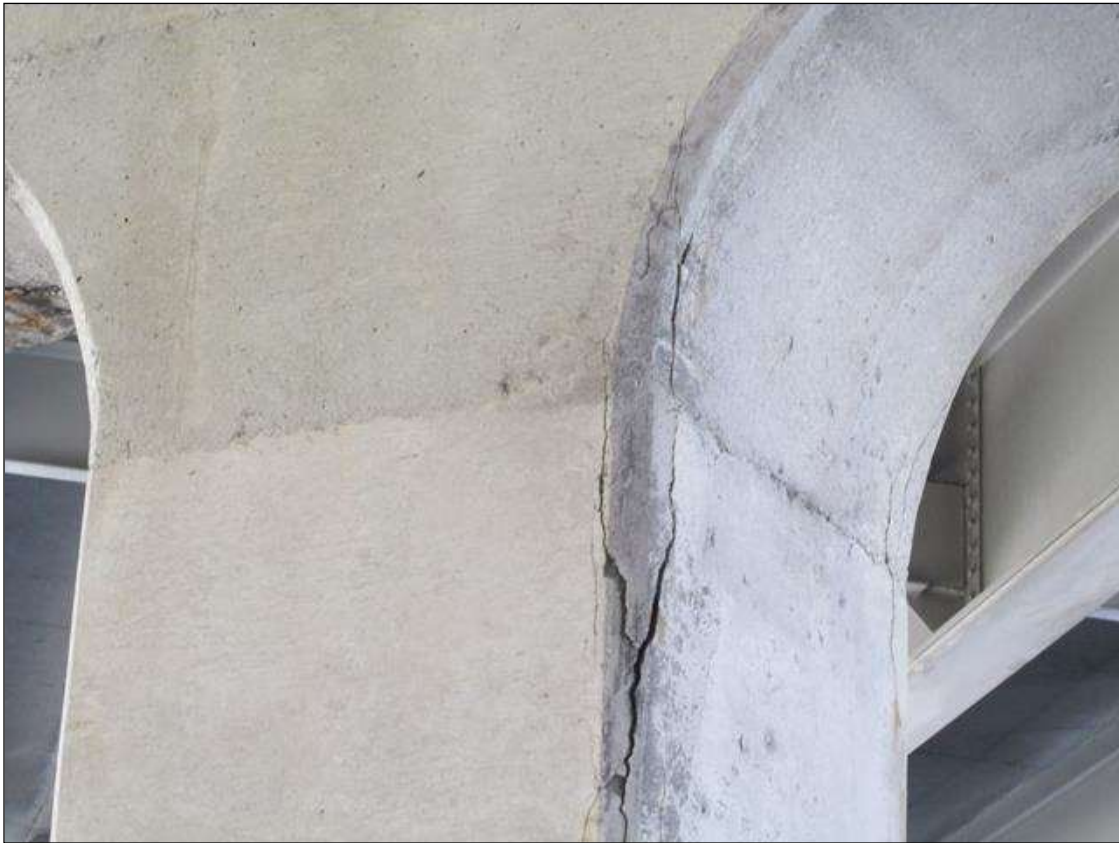
SPALLING, BENT 3, C3 RADIUS, APPROX 4'L
