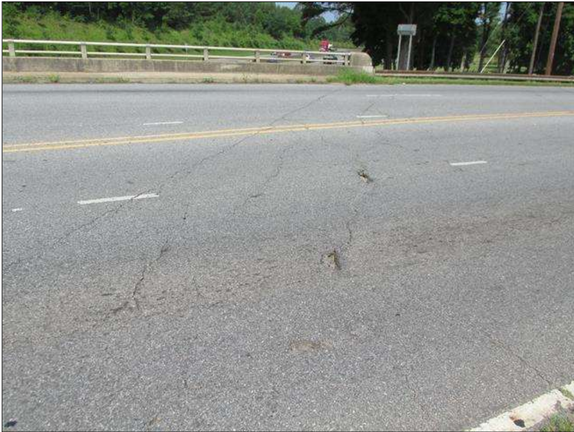
NORTH APPROACH AWS CRACKED, POTHOLED, AND SUNKEN UP TO 1.5", FULL WIDTH.
