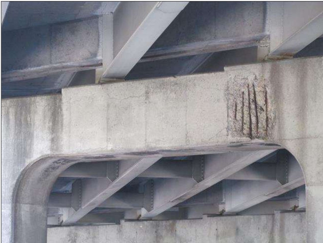
SPALLING WITH RESTEEL EXPOSED, BENT 2 CAP, BETWEEN C1-2 AND BETWEEN C2-3, TOTAL AREA APPROX 35SF
