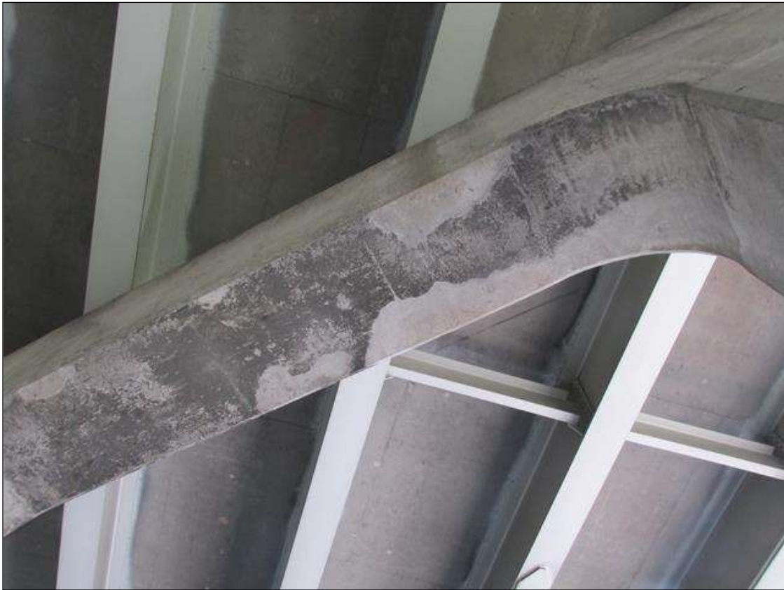
TEMP REPAIRS TO SPALLS SCATTERED ON BENT 1 CAP
