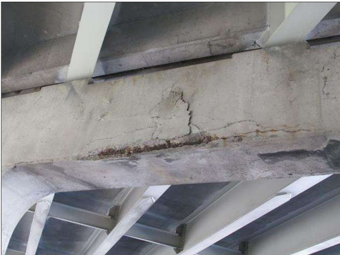
SPALLING WITH RESTEEL EXPOSED, BENT 3 CAP, BTWN C2-3, BOTTOM STRANDS OF RESTEEL EXPOSED AT N CORNER, APPROX 8'L X 3'H
